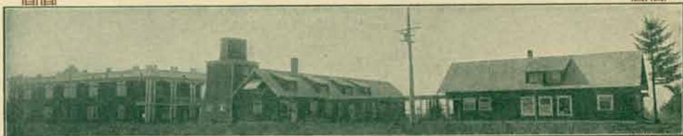
A row of buildings at Morningside
