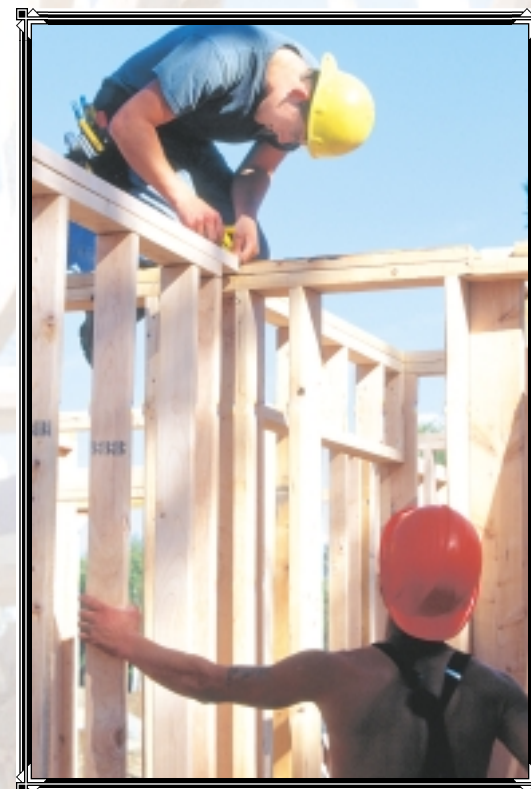
AHFC provided tax credits and long-term financing for the Ridgcrest Park Apartments, 40 units of low-income family housing in Wasilla, 42 miles north of Anchorage. The developer, Alpine Partners, is also constructing 32 units of senior housing on an adjoining property.
