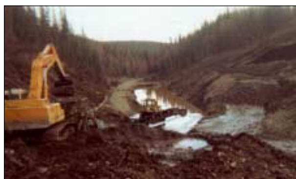
Figure 23. Looking downstream at Leo Regner's placer gold plant and settling ponds on Lilliwig Creek in the Fortymile area. Photo by Leo Regner.
