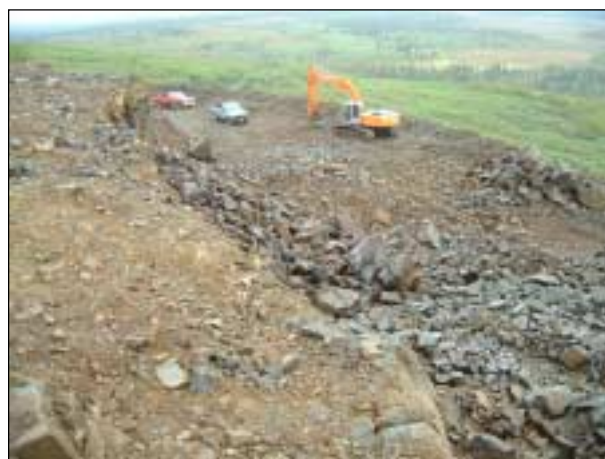
Figure 15. View of the new rock quarry 18 road miles from Dillingham that will provide a local source of material for various construction projects. Photo provided by Bristol Environmental and Engineering Services Corp.
