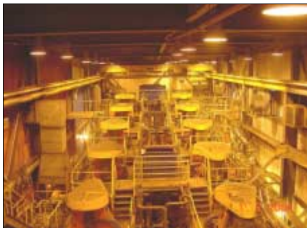
Figure 12. Newly expanded zinc circuit at the Red Dog mill. The zinc flotation module consists of 12 Outokumpu OK-50 flotation cells and four column cells (not shown). Photo provided by Teck Cominco Alaska Inc.
