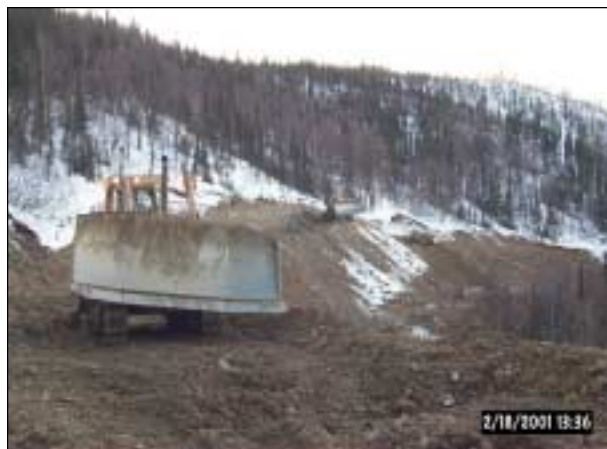
Figure 13. Fairbanks Gold Mining Inc. building a new road connecting the True North Mine to the Fort Knox Mine mill. Roadwork was completed during winter in steep terrain. Photo provided by Kinross Gold Corp.
