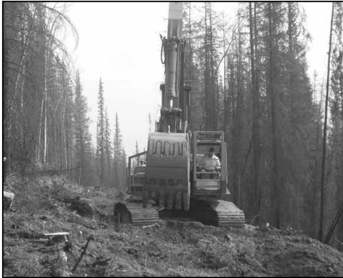
Delta Area road construction into the Camp Creek Fire Salvage Sale purchased by GIO Alaska Timber Corporation in August 2005. Photos by Steve Joslin.
