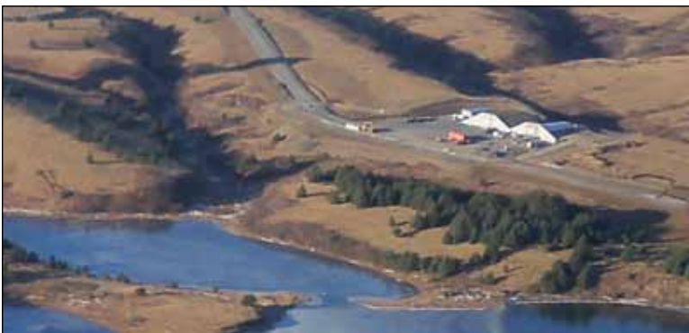
ECM1 and ECM2 at the Rocket Motor Storage Facility.
