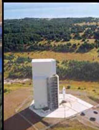
LAUNCH SERVICE STRUCTURE (LSS) AND LAUNCH PAD 1 (LP1)
