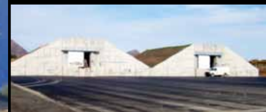
ROCKET MOTOR STORAGE FACILITY (RMSF)
