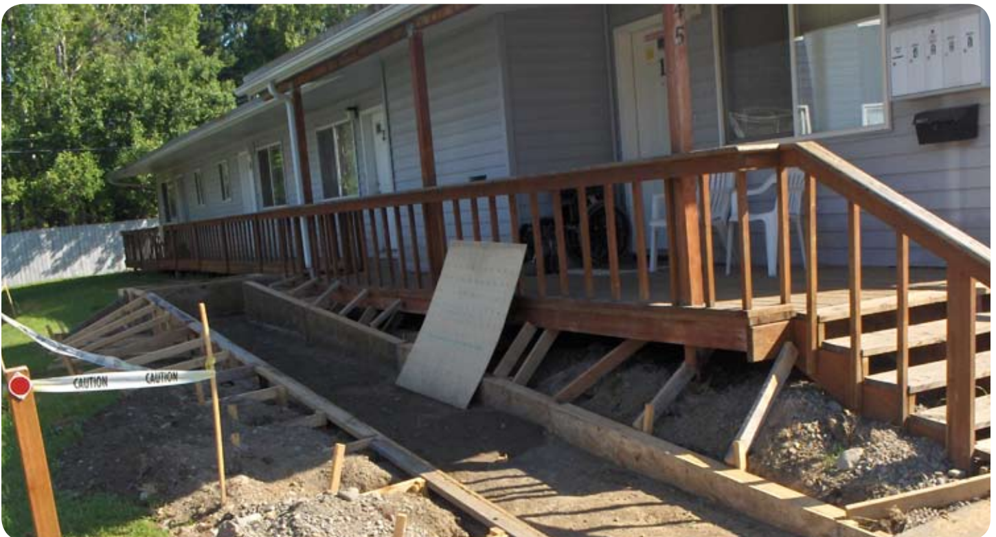
A handicapped-accessible walkway is installed at an Affordable Housing property in Mountain View
