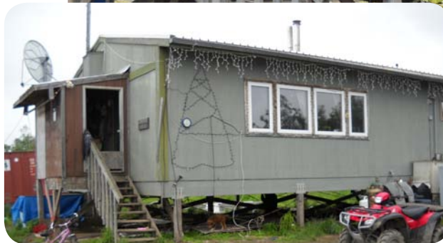
Before and after (top) weatherization of a home in Alakanuk.
