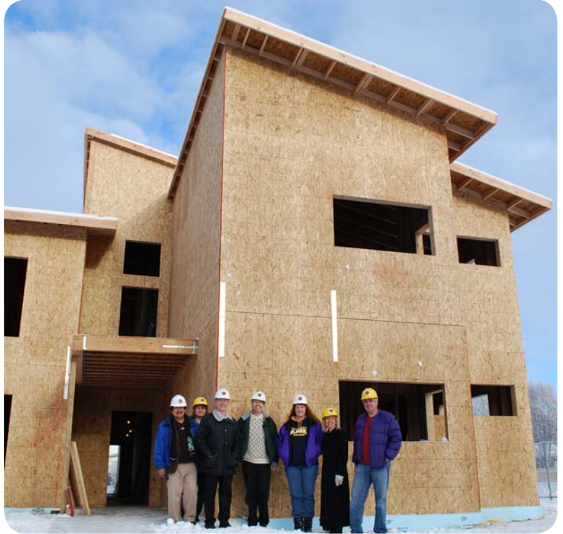
Board and staff members tour the new 7-plex Affordable Housing building in the Fairview neighborhood in Anchorage. Photo by Angela Gonzalez
