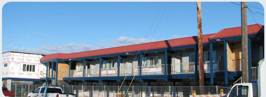
Karluk Manor during summer, 2011 renovations.
