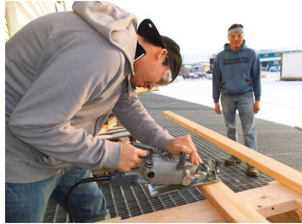
Martin Woods looks on as Instructor Tom Borce cuts wood in an Energy Wise training in Kotzebue. Energy Wise crew members receive Weatherization Tech 1 and OSHA 10 certifications.
