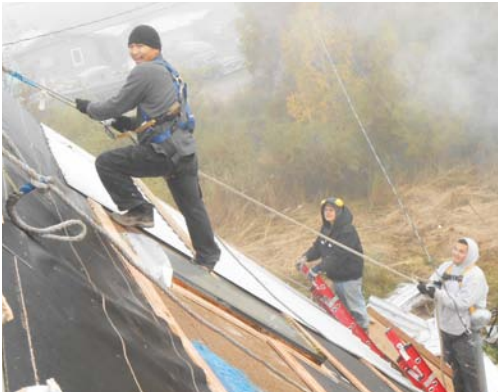
Weatherization workers insulate a roof of a home in Lower Kalskag.
