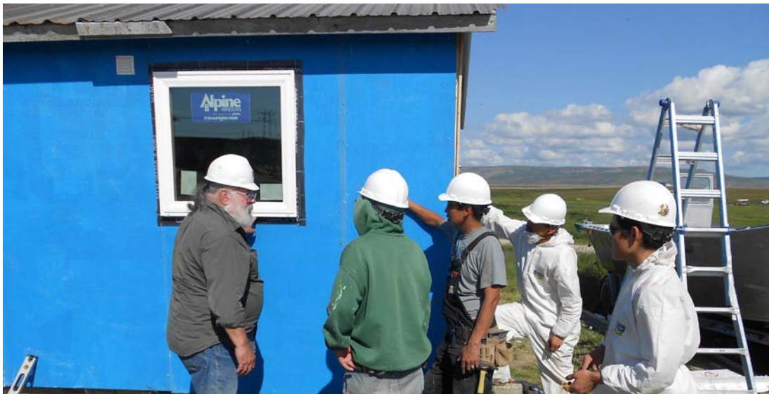
Mark Lyman (at left) teaches crew members in Toksook Bay about proper window insulation. Photo by Keith Perry
