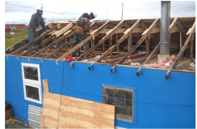
The Weatherization crew repairs a roof in Chevak. Photo courtesy of RurAL CAP staff
