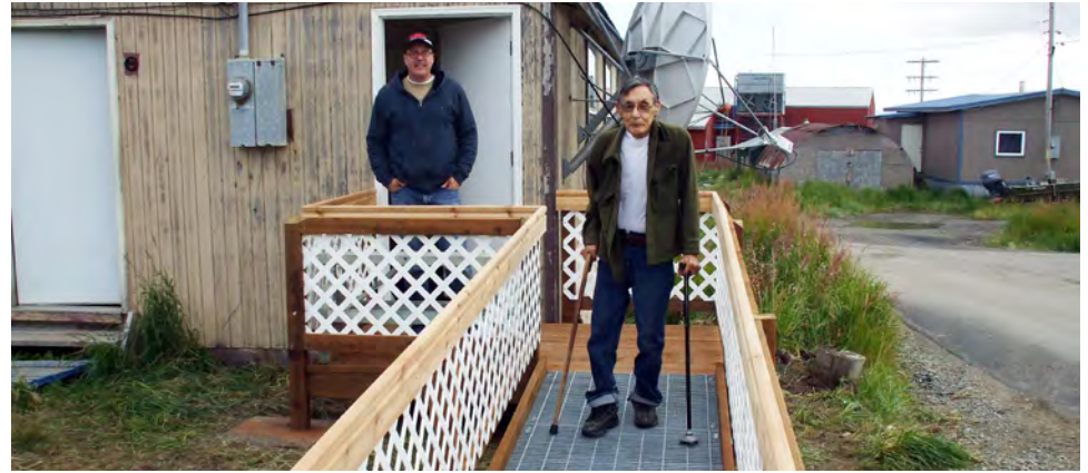
Irwin Barr of Unalakleet receives an entry ramp for his home through the Home Modification program. Barr is pictured with Jon Liebsack of RurAL CAP. Photo by Sam Meyer
