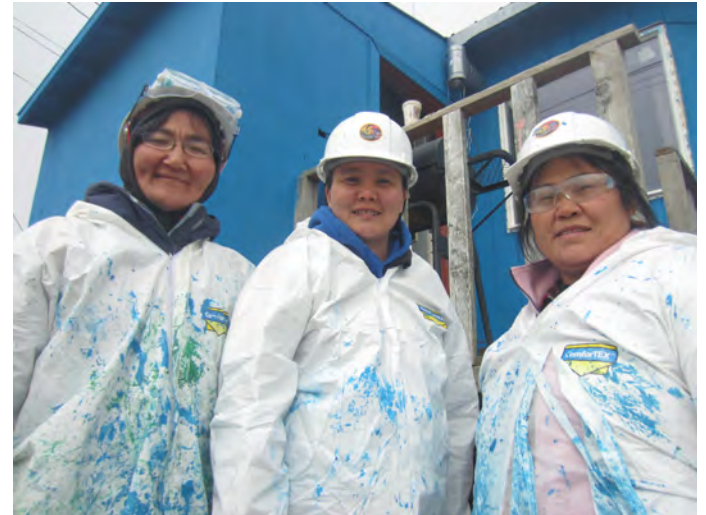
The weatherization crew paint homes in Toksook Bay.
