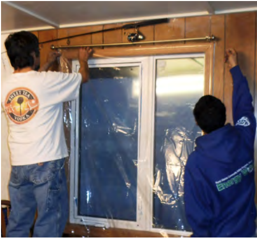
Energy Wise crew members seal a window in Deering to increase energy efficiency.
