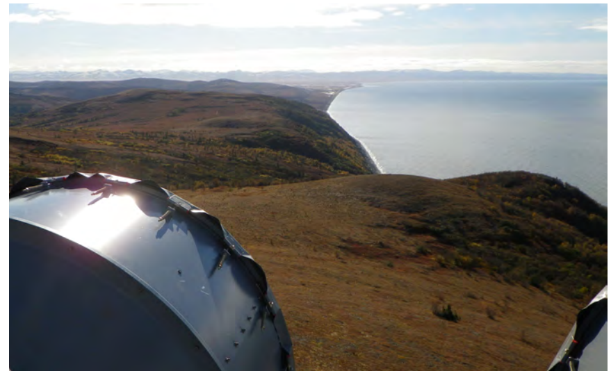
Unalakleet mountaintop repeater view from above. Photo courtesy of GCI
