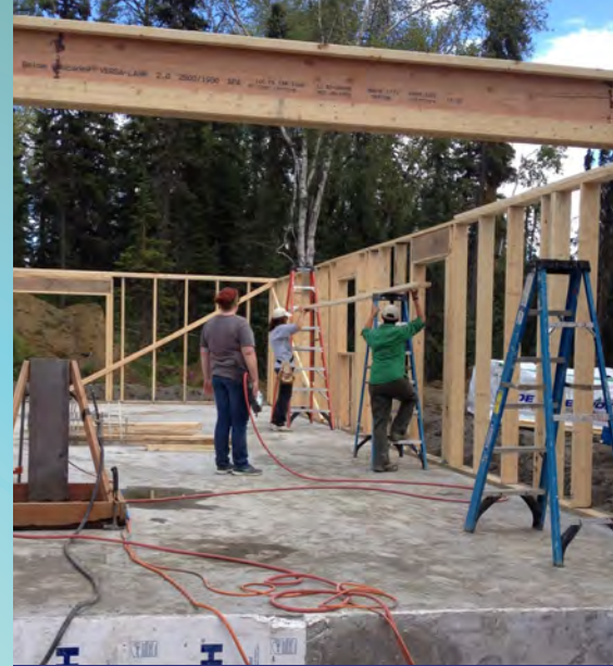
Homeowners and volunteers help build Self-Help homes on the Kenai Peninsula. Photo by Mi'shell French
