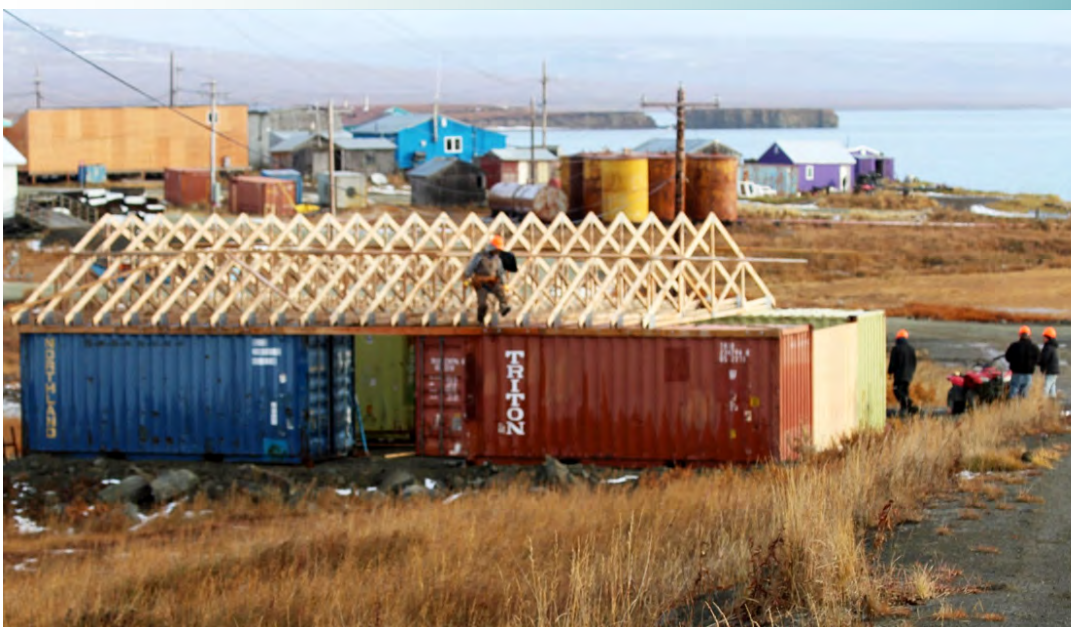
An e-waste and equipment storage building under construction in Toksook Bay for a solid waste project. Photo by Ted Jacobson
