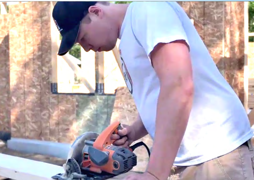
A Self-Help Housing homeowner, Ryan McMilin, helps build his home in Soldotna. Photo by Charlie Ess
