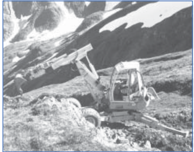
A "Menzi muck" machine carves out a trench to bury power lines. Photo is courtesy of Alaska Electric Light & Power Company.
