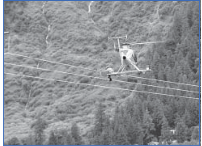
A helicopter crew replaces old aircraft marker balls on the 69kv transmission line in Juneau. Photo is courtesy of Alaska Electric Light & Power Company.
