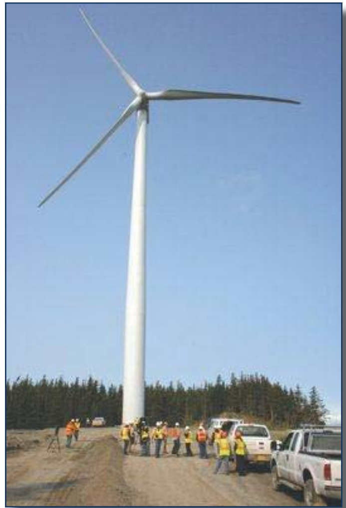
Fire Island Turbines are now providing power to the South Central Ratepayers.
