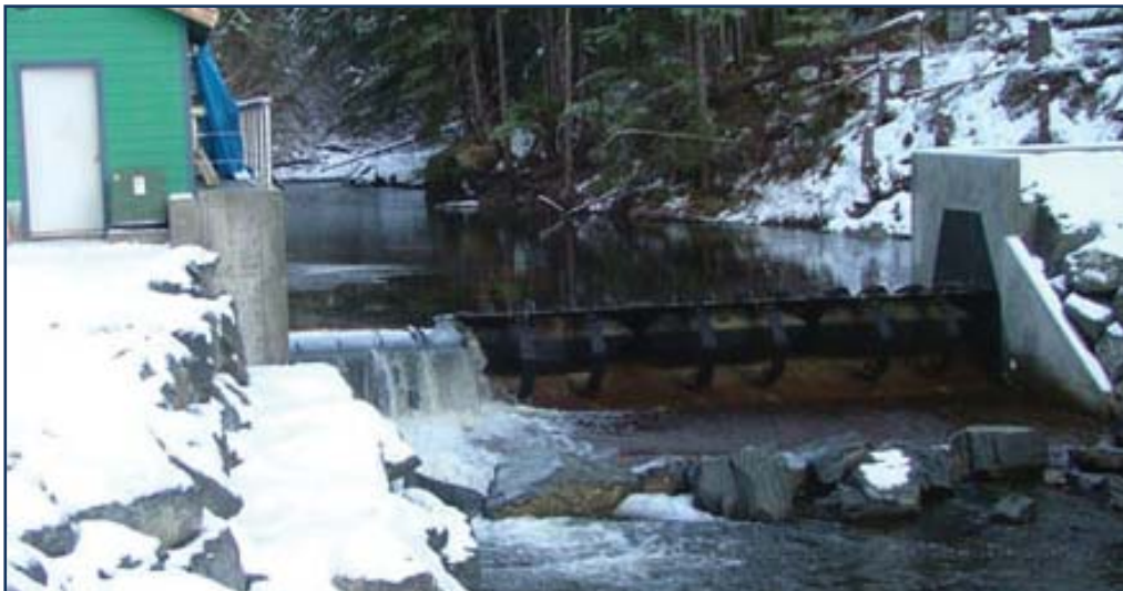
Falls Creek hydroelectric power project serves the community of Gustavus
