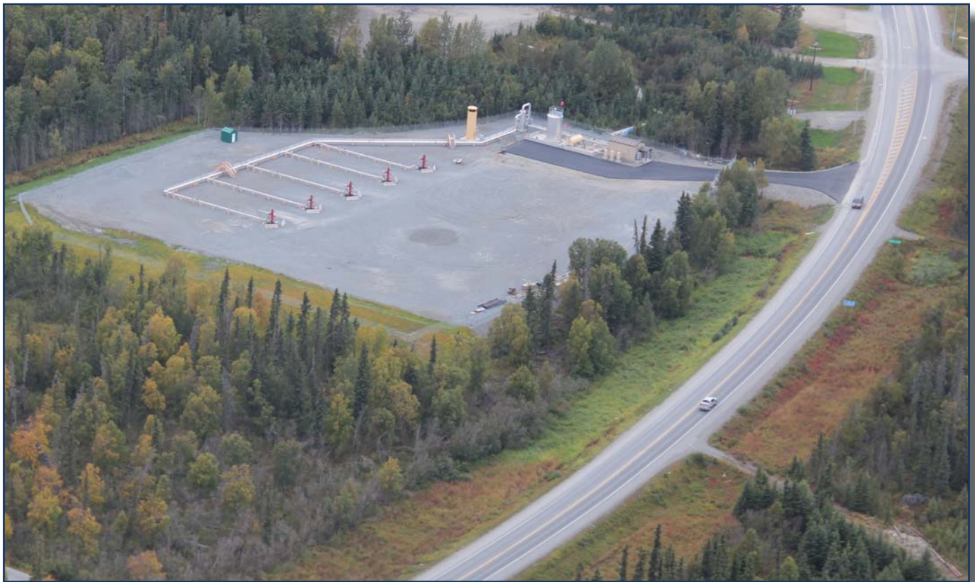
Cook Inlet Natural Gas Storage – Alaska. An aerial view of the storage facility operations pad located in Kenai Alaska.
