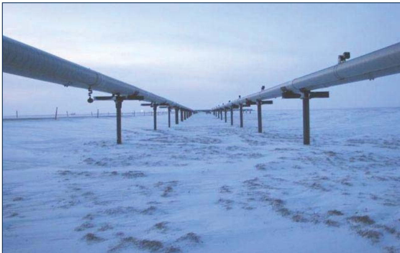
Milne Point pipelines VSM 222 to VSM 432.
