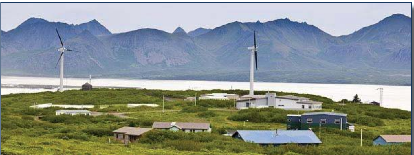
TDX Power Turbines in St Paul.
