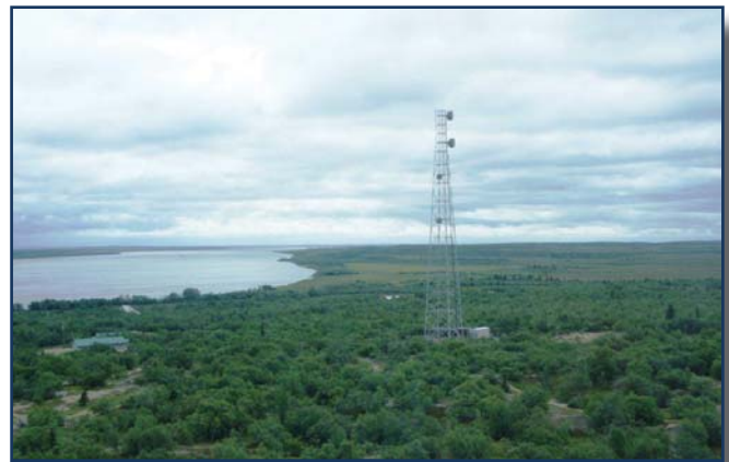
Microwave Tower in Levelock – Enhancing telecommunications in rural Alaska.
