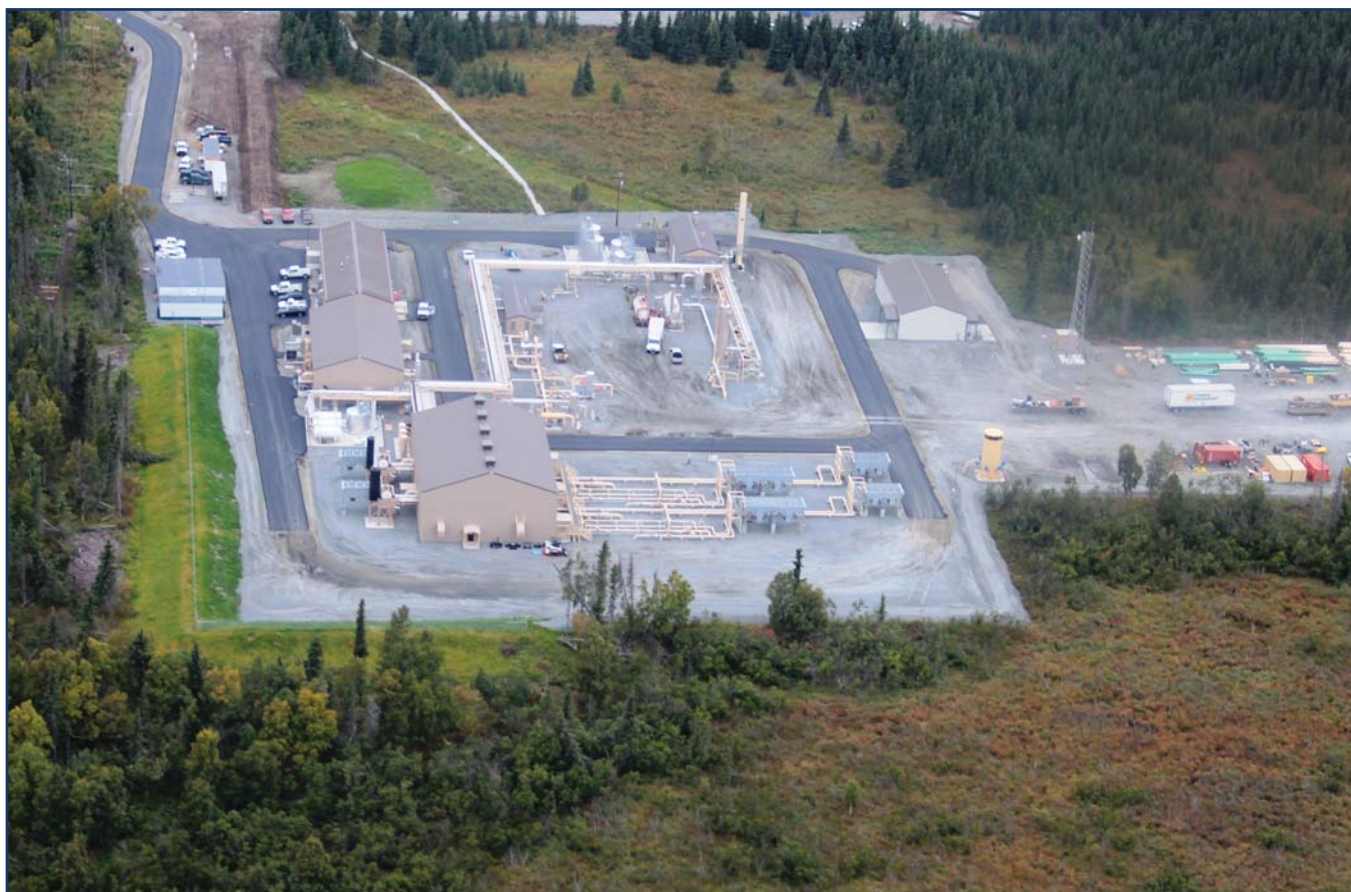
Cook Inlet Natural Gas Storage Alaska – an aerial view of the facilities located in Kenai Alaska.
