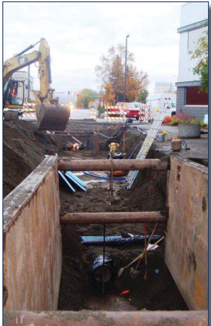
AWWU work in progress in the Spenard area of Anchorage.
