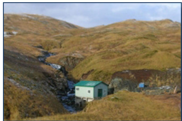
City of Atka's Chuniisax Creek Hydro Station
