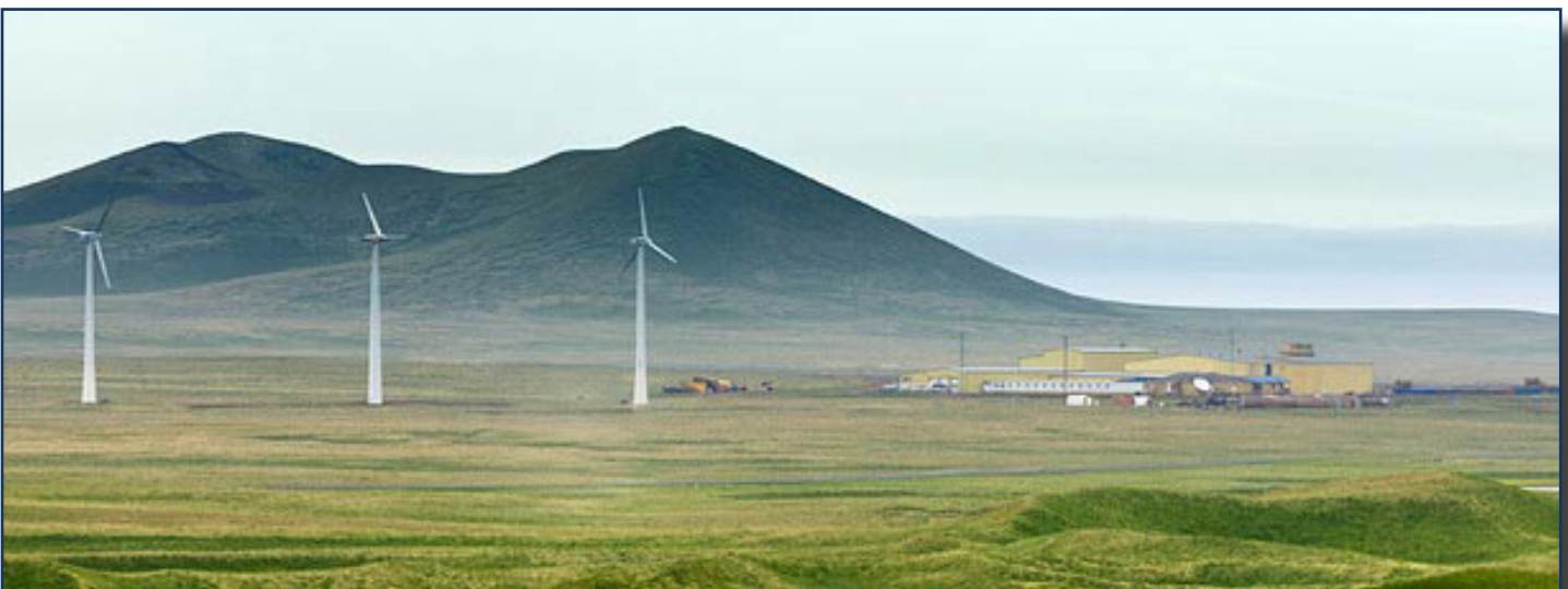
TDX Power turbines
