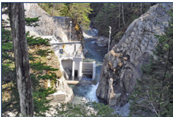
Cordova Electric Cooperative's Humpback Creek Hydro Station
