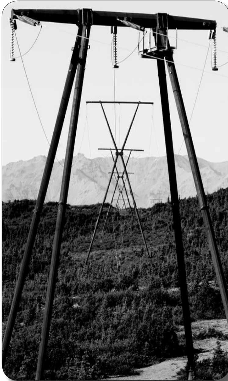
A section of the Alaska Intertie, built in the 1980s, stretches out near Healy.
