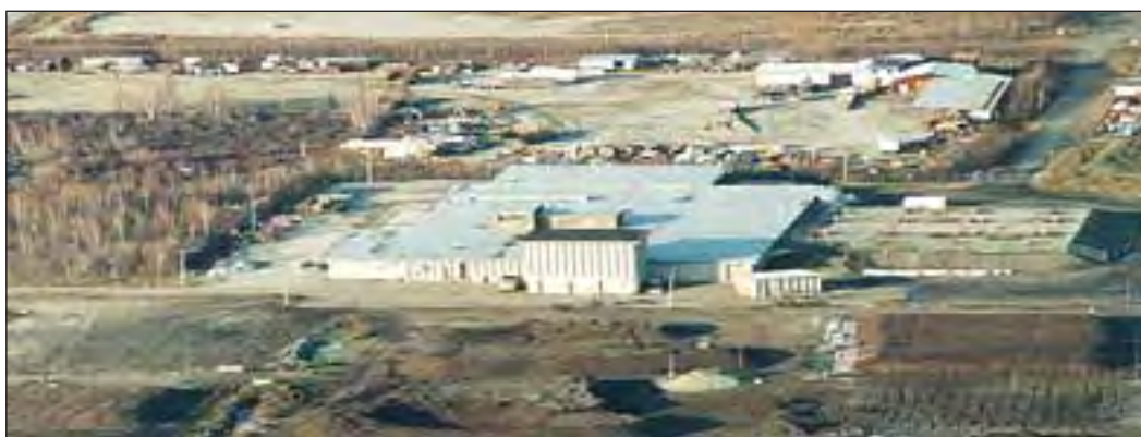
Aerial view of Golden Heart Utilities/College Utilities Wastewater treatment plant.
