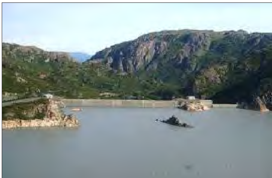
The dam at Bradley Lake.
