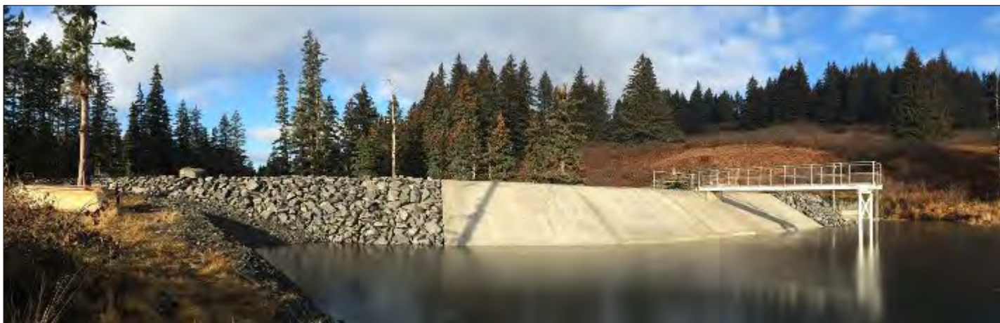
Pictured Above is the newly completed Ouzinkie Dam. The new dam was completed in 2014 replacing an aging wooden structure. The project is part of Alaska Native Tribal Health Consortium's Rural Energy Initiative. Photo Courtesy of ANTHC.
