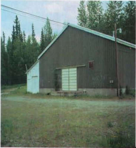
Vandalism at the Geologic Materials Center June 7, 2007
