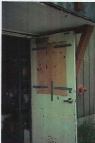
Front door and window
