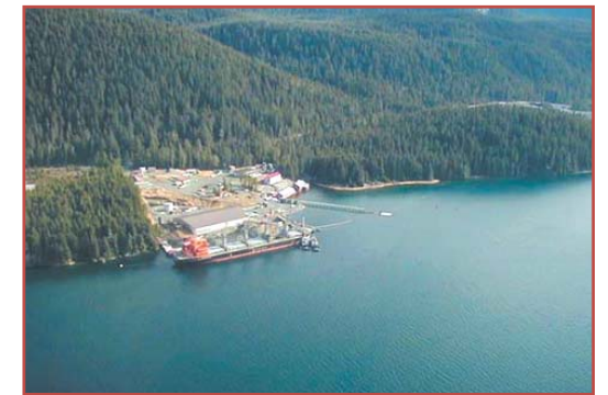
Greens Creek Ship Loading.
