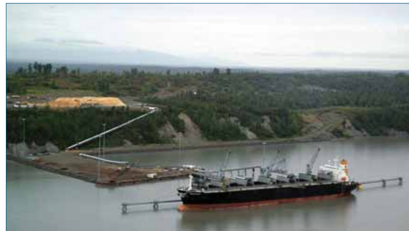
The Keoyang Majesty used Port MacKenzie's newly completed deep-draft dock to load wood chips bound for Korea in February 2005. In 2005 six panamax size vessels and twelve barges used the new dock; it can accommodate panamax and cape sized vessels and ships with drafts up to 60 feet. Photo courtesy of Port MacKenzie
