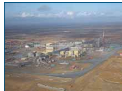
VECO partnered with Eastern Construction Company on the Chayvo oil production facility on Sakhalin Island, Russia.
