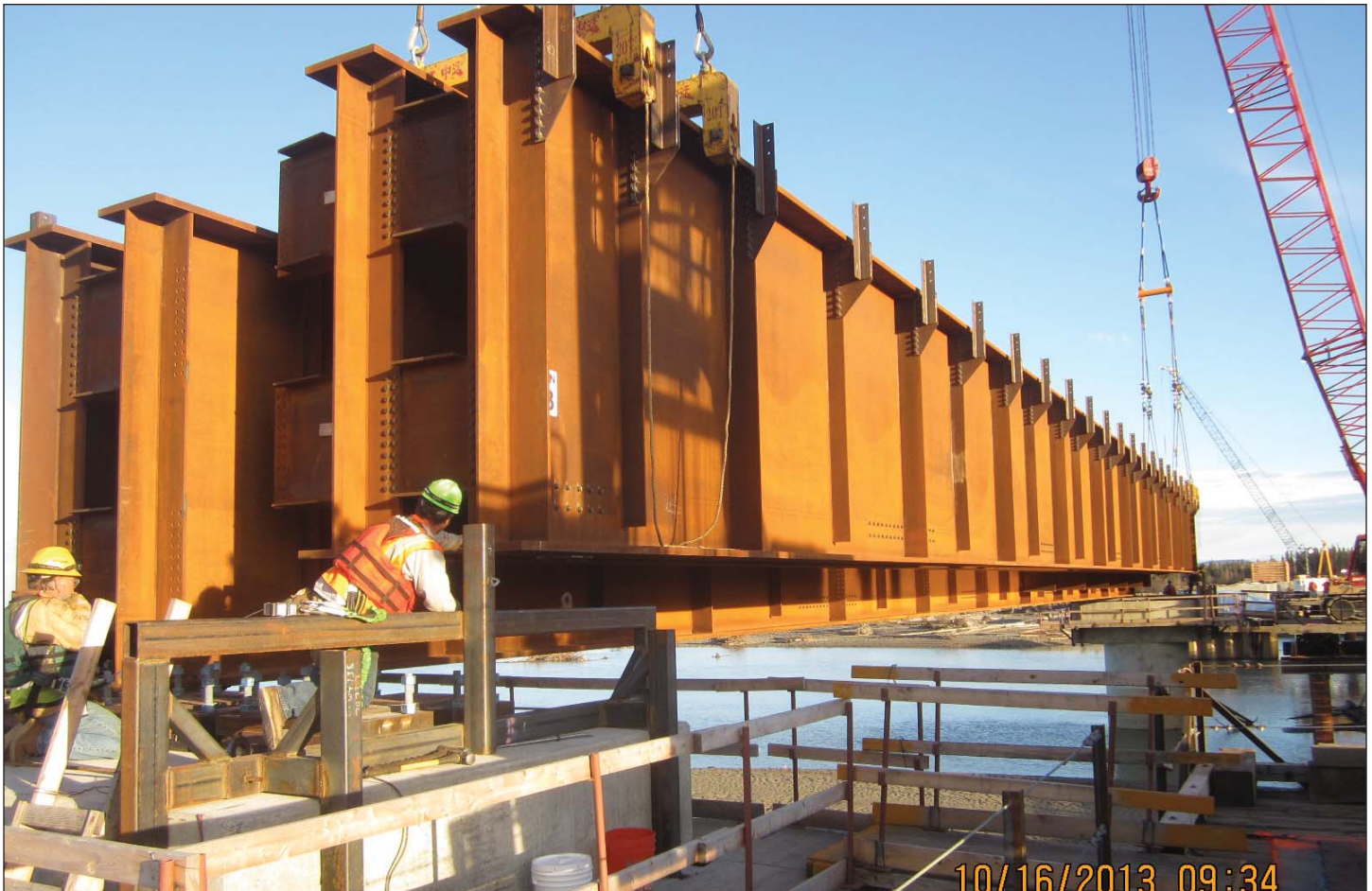
Above: The first span of 165-foot girders are placed on two piers as part of the Northern Rail Extension (NRE) Phase 1, the Tanana River bridge near Salcha. Cover top photo: Construction on the NRE Phase 1 bridge stretches across the Tanana River in early November 2013.
