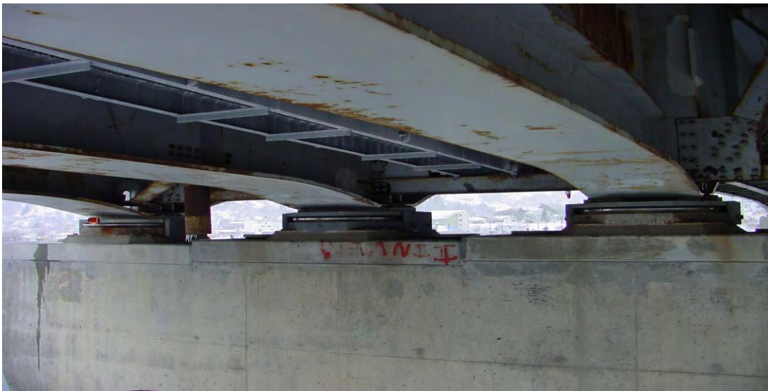
Figure 10. Seismic Retrofit using Friction Pendulum Bridge Bearings, Kodiak Harbor Channel Bridge
