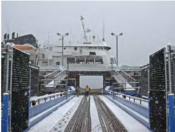
Figure 18. Ferry Terminal Ramp
