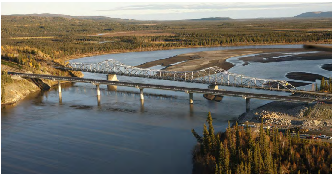
Figure 15. New and Old Tanana River Bridges
