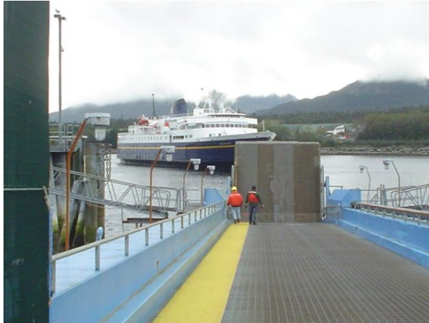
Figure 19. Ketchikan Ferry Terminal Ramp
