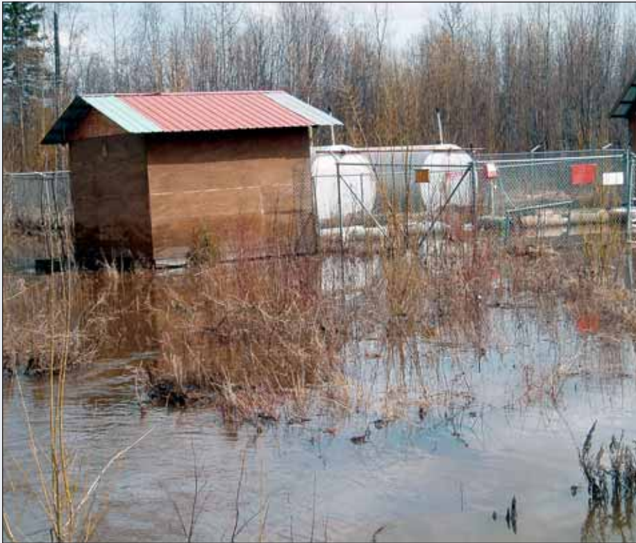
Propane Tanks Problems. Flood waters affected infrastructure components in communities, such as the propane tank farm in Koyukuk. Photo: Kerry Seifert, DHS&EM
