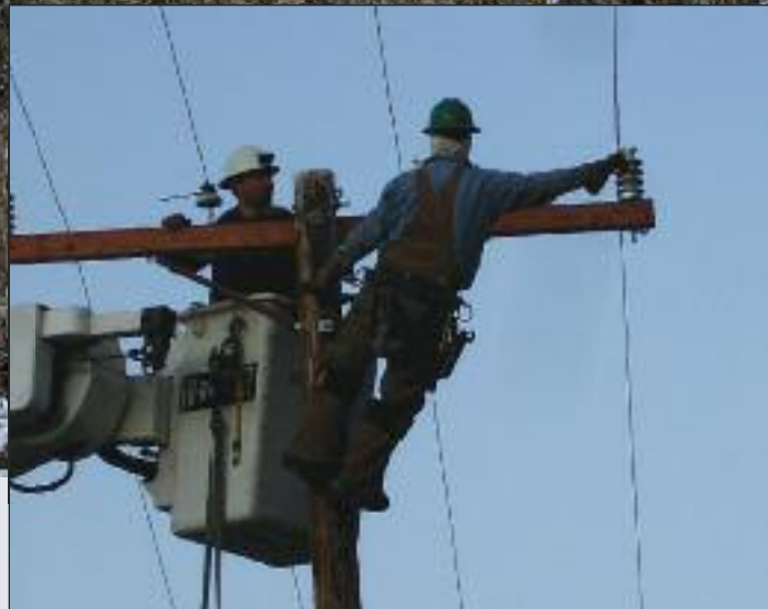
Damage Repairs. Linemen with Homer Electric Association repair damaged power lines along the Kenai Peninsula after November windstorms left approximately 17,300 homes and businesses without power for as much as 48 hours.
