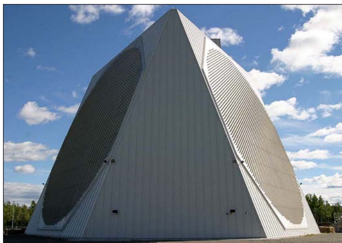
SSFARS Radar Clear Air Station. A Solid State Phased Array Radar System radar in a protective dome stands 11-stories tall on Clear Air Force Station. The station's primary duty is to provide an early warning of intercontinental ballistic missiles and submarine-launched ballistic missiles. Photo: Courtesy of 213th Space Warning Squadron
