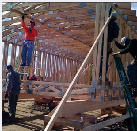
Volunteers Frame First New Home. Skilled volunteers complete the framing in one day using designs and materials customized for Crooked Creek.
