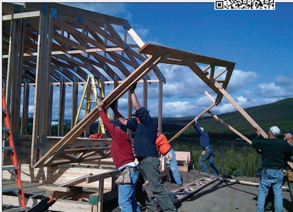
Team Work. Samaritan's Purse and Christian Reformed World Relief Committee volunteers work together to erect pre-engineered housing components.
