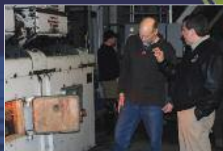
Senator Tours Clear Air Force Station. Leroy Sutton, operations and maintenance supervisor, 213th Space Warning Squadron, left, briefs U.S. Senator Mark Begich on the operation of Clear Air Force Station's power plant in April. Begich toured the facilities at Clear Air Force Station, about five miles south of Anderson, Alaska, and learned about issues facing Clear, upcoming military construction project requirements, and the radar's current capabilities and funding targets for the upgrade.
