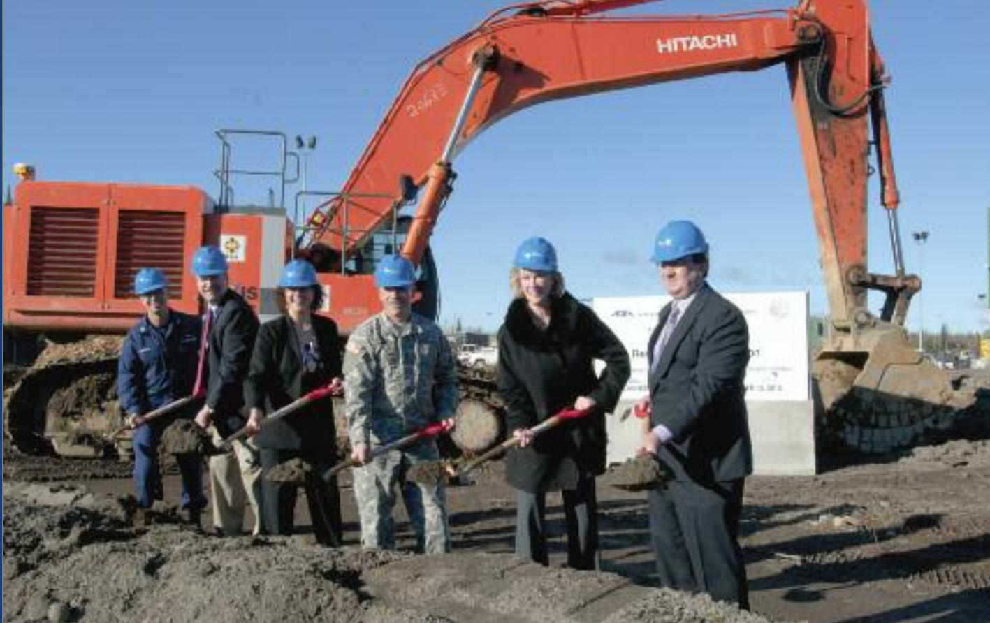
Total Force Integration Ground Breaking. From left, Shane Montoya, U.S. Coast Guard; Representative Dan Saddler, State House of Representatives; Commissioner Susan Bell, Department of Commerce, Community and Economic Development; Major General Thomas H. Katkus, Department of Military & Veterans Affairs; Nancy Dahlstrom, Office of Governor Sean Parnell; and Al Luck, Joint Base Elmendorf-Richardson, ceremoniously break ground in October on the new Alaska National Guard Armory G Wing on Joint Base Elmendorf-Richardson. The new wing is scheduled to be completed in December 2013. Photo: Staff Sergeant Karima Turner, 134th Public Affairs Detachment
