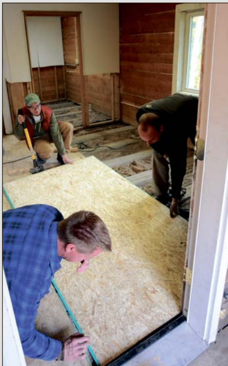
Volunteers at Work. United Methodist Volunteers in Mission replace flooring and insulation last summer in Galena. Through the tremendous effort of volunteers almost all residents were able to return to their homes prior to winter. Photo: Brock Jones, DHS&EM
