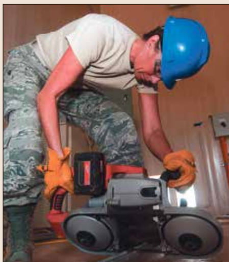
Power Cuts. Master Sgt. Bonnie Gardino, utilities supervisor for the Alaska Air National Guard's 176th Civil Engineer Squadron, cuts structural support braces at a small outpost in Australia during a Deployment for Training in May.
