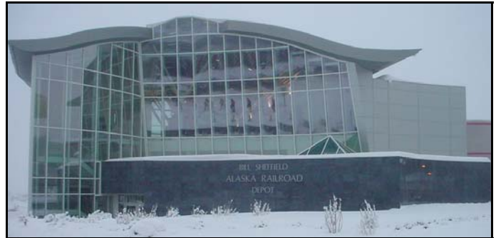
BILL SHEFFIELD ALASKA RAILROAD DEPOT LOCATED AT ANCHORAGE INTERNATIONAL AIRPORT
