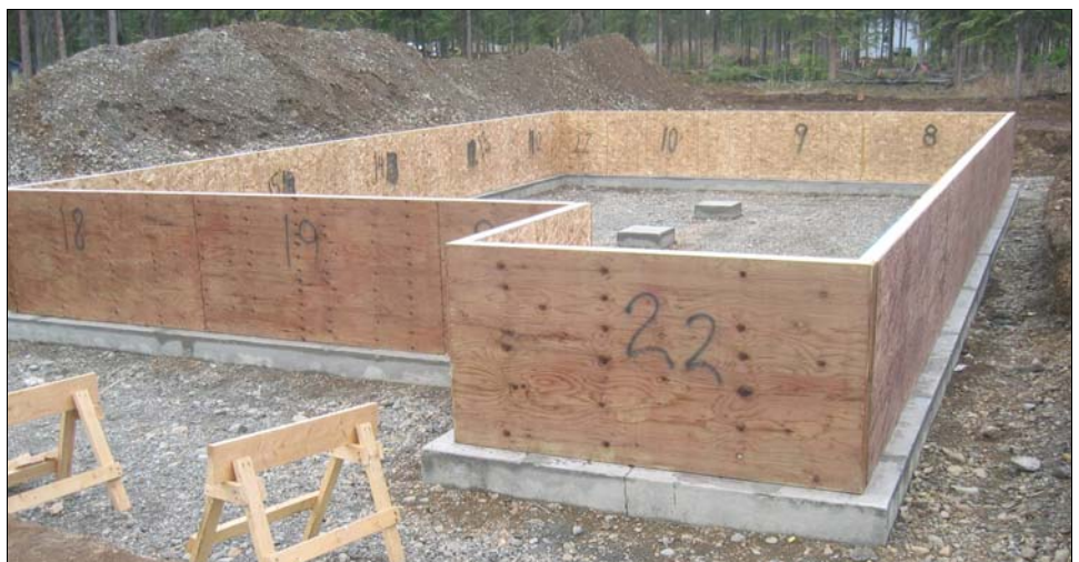
Foundation on one of the houses
