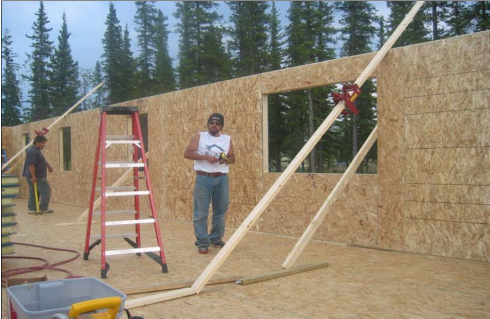
Work on one of the houses
