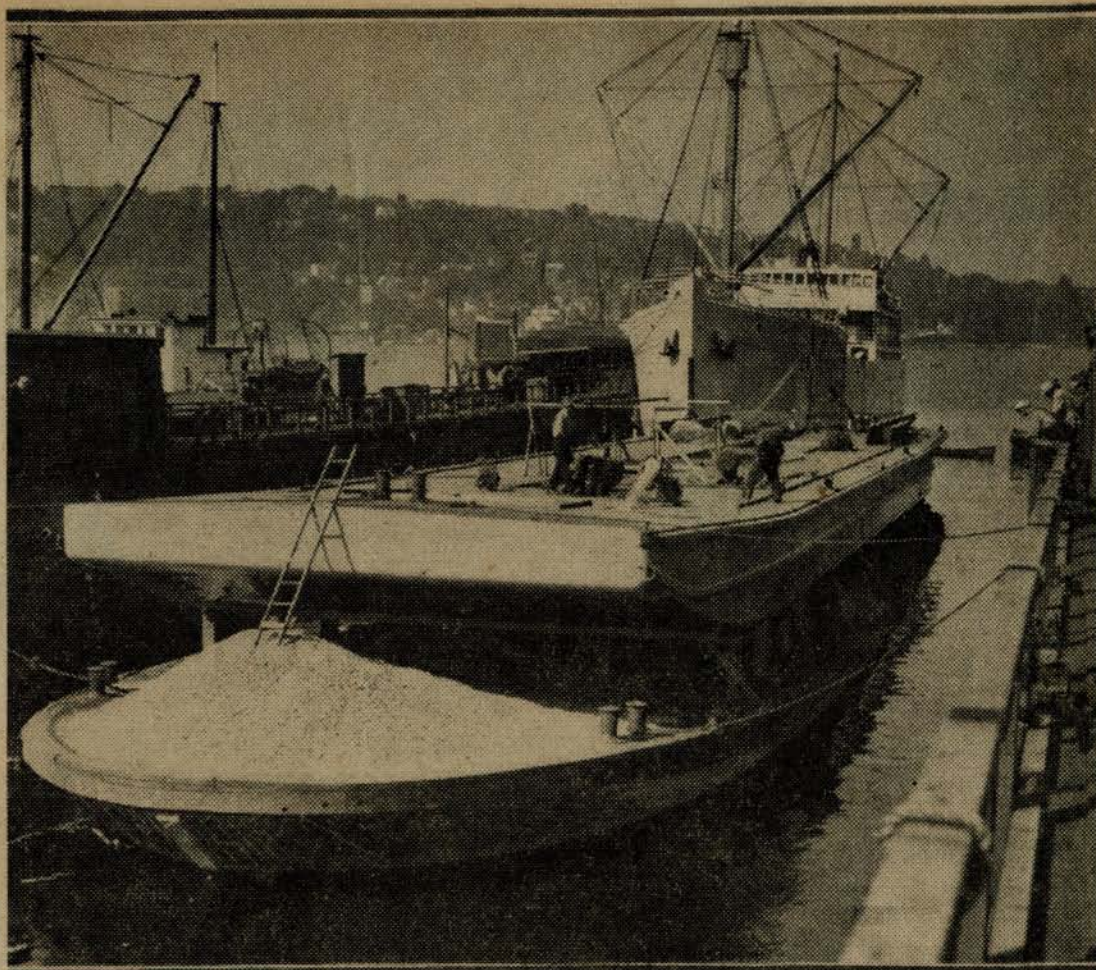
The steel hull of the United States Army Engineer Corps' new "snagboat" was floated yesterday at the Lake Union Drydock. The hull was built on a barge and took to the water where the barge was submerged by being filled with water and ballast. The boat will be under construction six weeks more at the Lake Union yards. This picture shows the new hull on the barge just before the latter was submerged in new-fashioned launching procedure.
